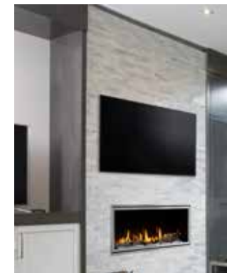
Passive Heat Open Wall Register (opening 2" from ceiling)
